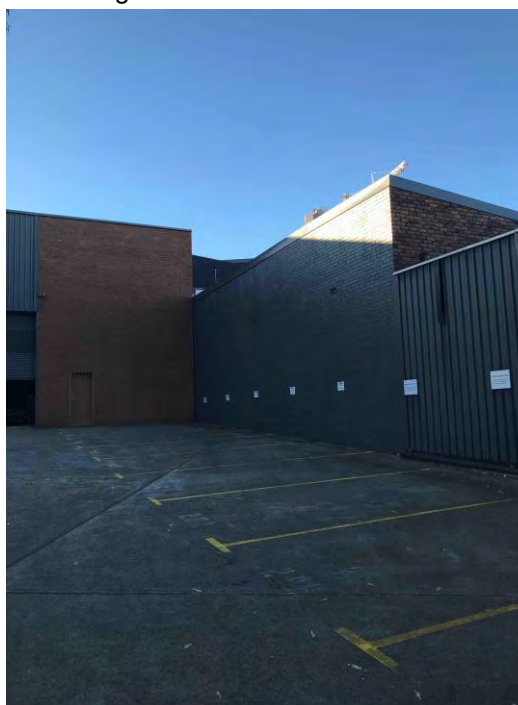
Photo 2: Car park in far south west area of the site.
